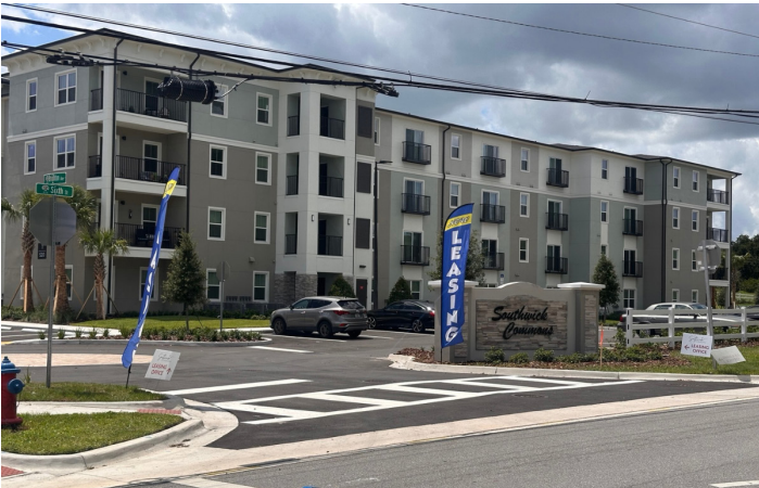
Southwick Commons, a 192-unit affordable housing development at 520 Brighton Ave. in Apopka, is now open and leasing one-, two- and three-bedroom apartments. | PHOTO BY TERESA SARGEANT
