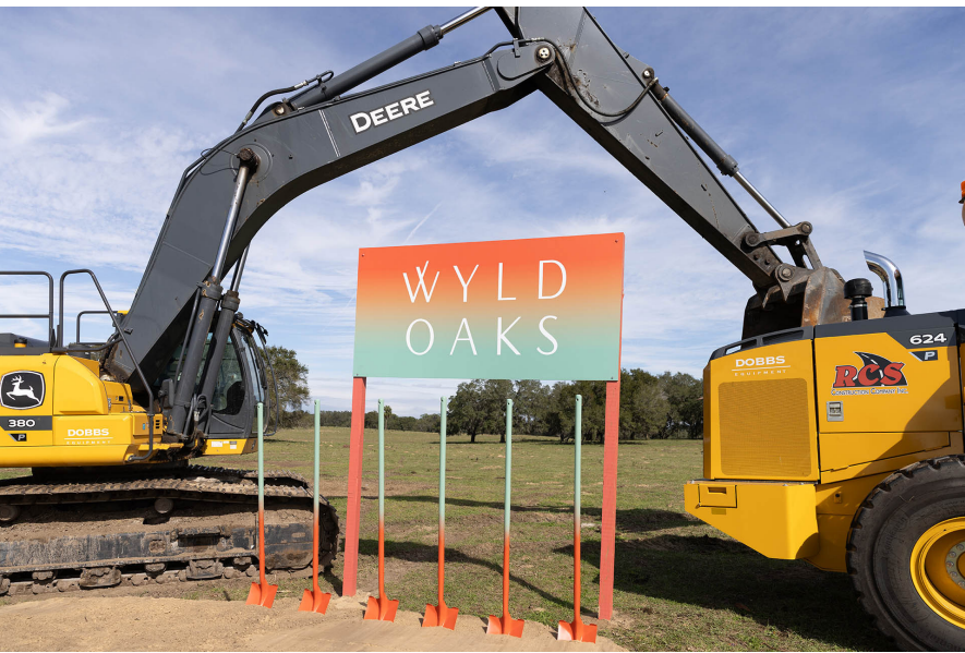
Construction equipment is shown at the Wyld Oaks development in this promotional photo. The Apopka Development Review Committee reviewed the first construction site plan submittal Wednesday for an approximately 600-foot extension of Road C within the development. | COURTESY OF WYLD OAKS
